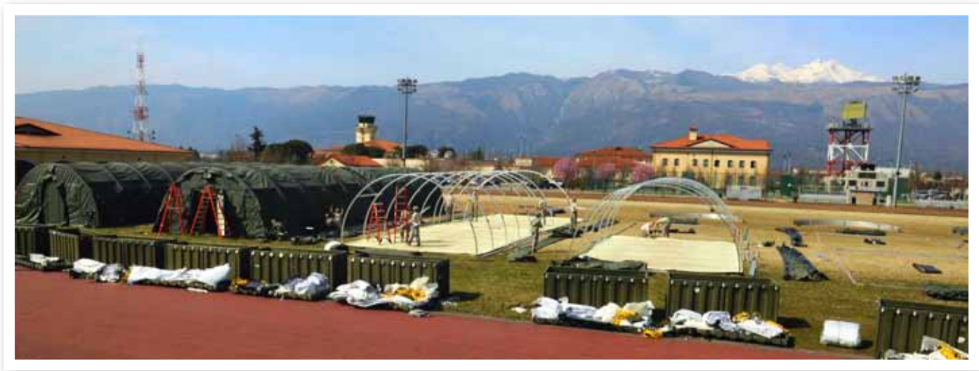
31 FW/JA - Aviano OUP tent city under construction
